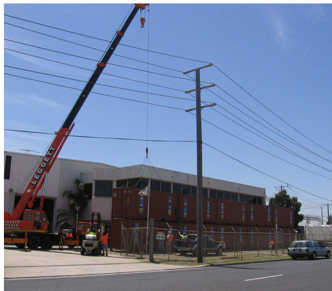
Figure 6 Shipping Containers Being Placed to Control LFN
